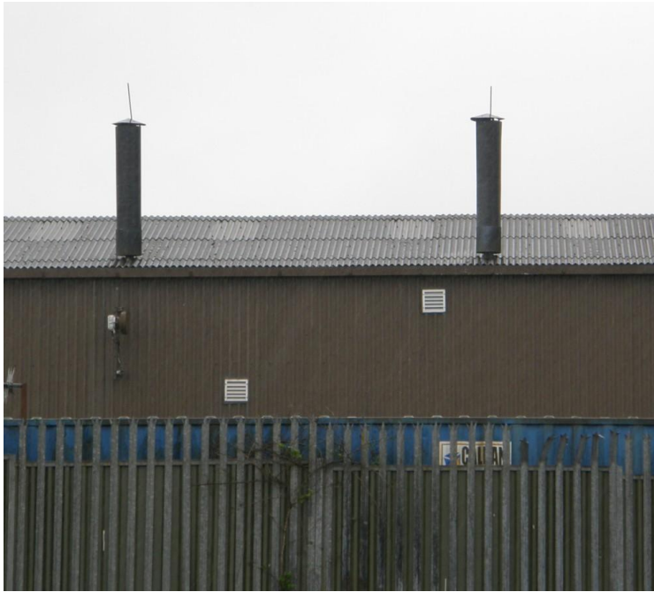
Transmitter Site Photo
